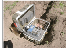
3- The recording unit is placed in hole and connected to solar panels and battery
