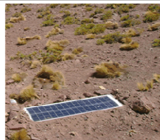
4- After installation, only the solar panel is visible on the surface
