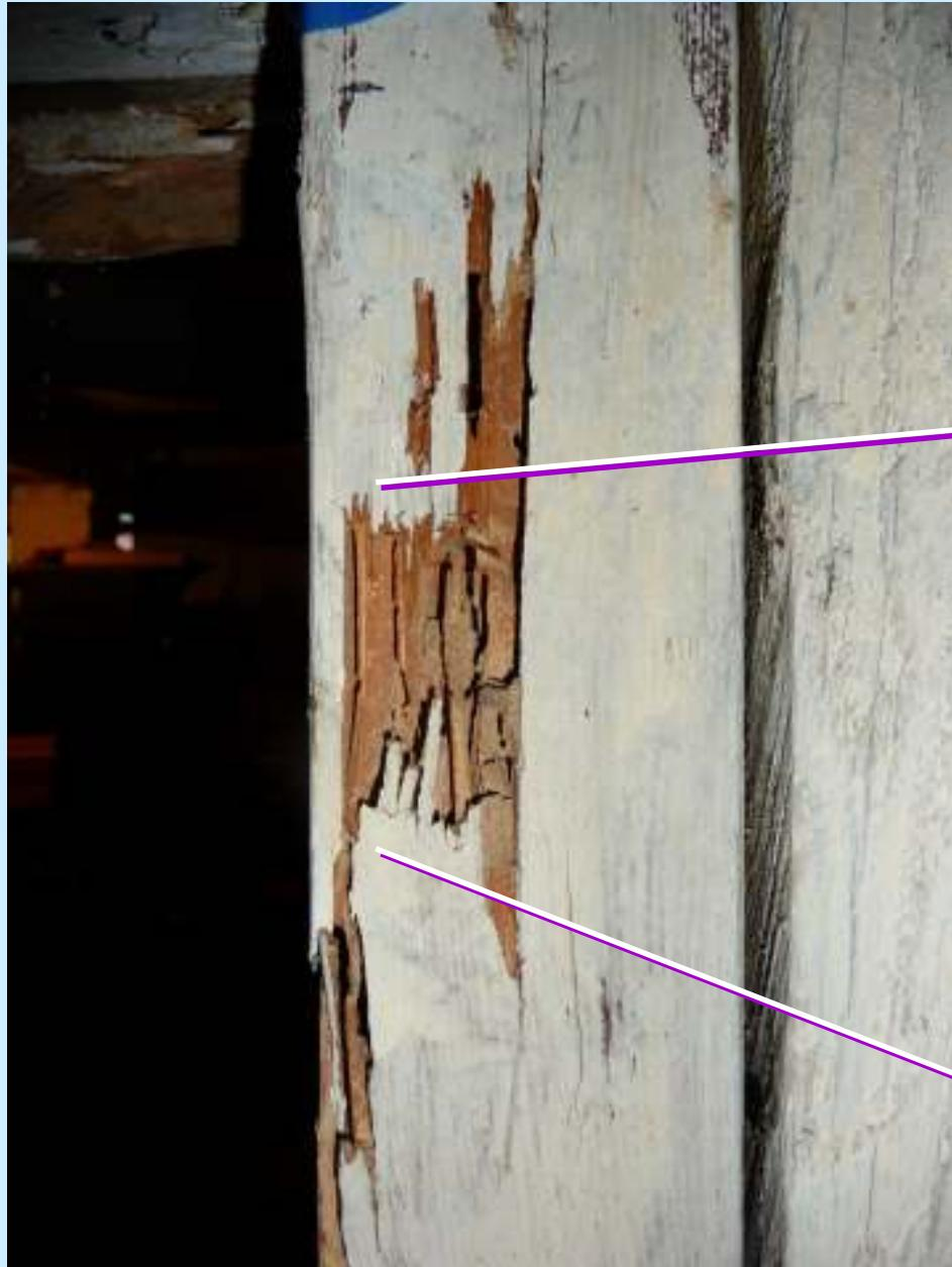
The Radar anomaly was probed with a screwdriver, revealing hidden tunnels.
