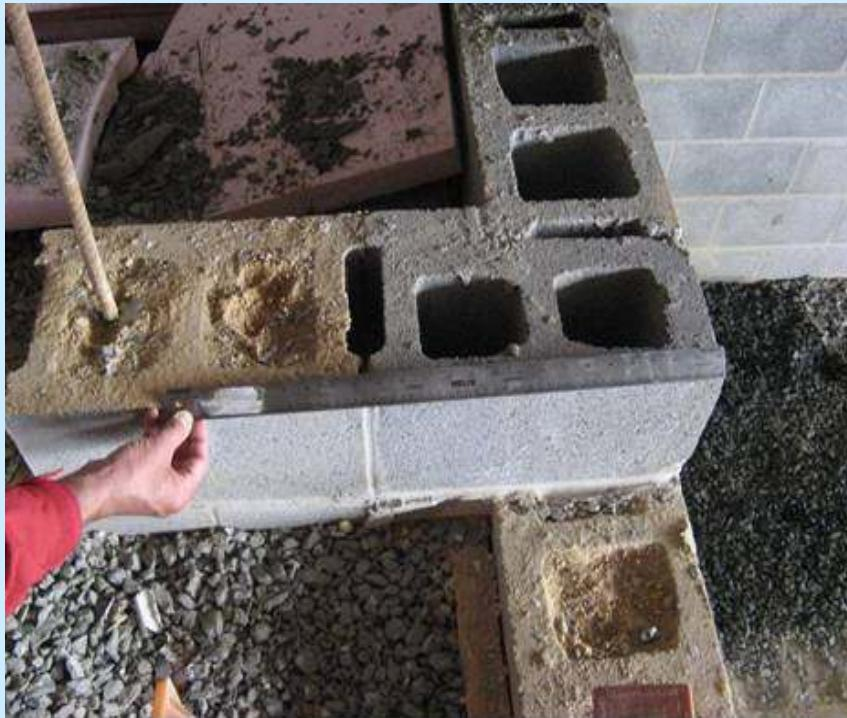
Concrete blocks with dimensions about  $40 \times 24 \times 20\text{cm}^3$ . The internal part of the blocks has two holes of  $12.5 \times 16\text{cm}^2$
