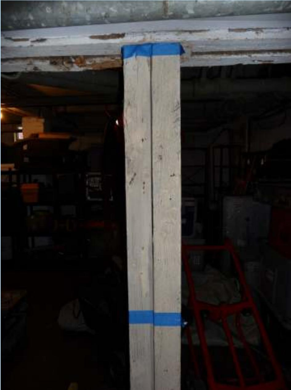
This double post shows no visible surficial damage, but the beams above do.
