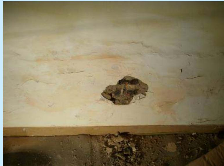
The section of the original bricks (about 100 years old) has dimension 28 cm x 4 cm , separated by mortar with thickness of about 2 cm. The plaster coating has a thickness of 1.5 cm for area #1 and about 3 cm in the lower moisten area
