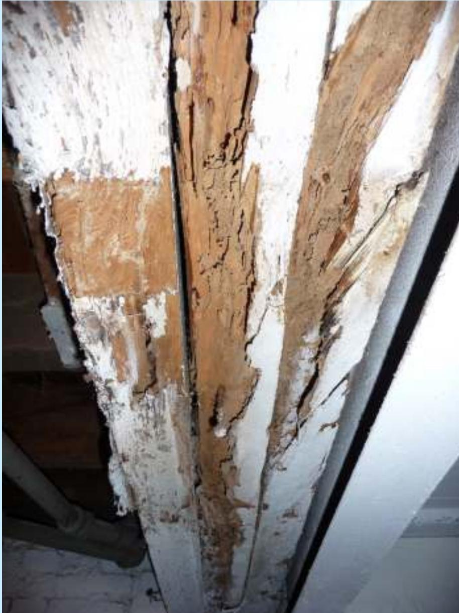
Radar was used in a building with heavy termite damage, from an old (>10 years ago) infestation.
